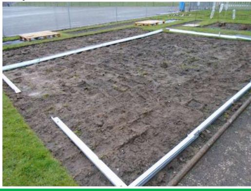
On the left you can see the steel base has all been set out before it is all fixed together.. From this base the rest of the framework is then assembled.....
