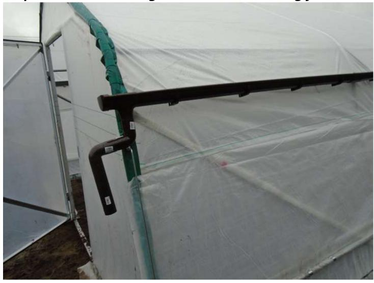
Guttering to both sides is being fitted which will feed into two water butts that we are going to set up – with the surface area of the poly tunnel being a considerable space, it will allow the capture of a significant amount of water – excellent for watering our crops plus environmentally friendly too.....
