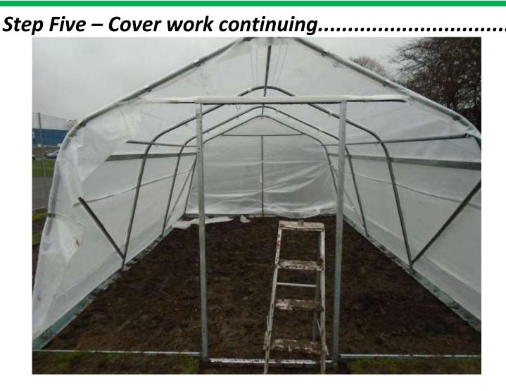
Above you can see that the back end of the poly tunnel has now been covered so the coverage of the tunnel is getting closer to completion.....
