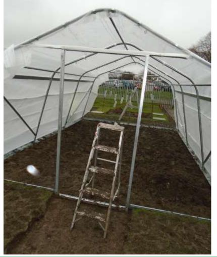
Now that the steel framework has all been set up – now is the time to start to put the cover over the framework to create our indoor poly tunnel space...... As you can see the cover goes on in sections with the main section going on first which is then securely fastened before the back and the front sections are added..
