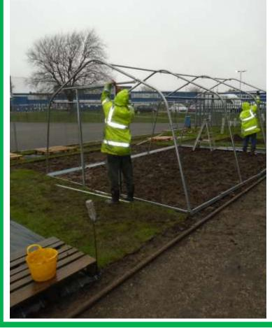
On the left you can see the continuation of the framework set up with the door frame assembled ready and in position.... Once the steel framework has all been fitted together, the whole structure is fixed into the ground with steel posts to give it excellent ground anchorage... A vital component of the poly tunnel set up especially bearing in mind some of the extremely high winds we have been experiencing in recent times.....
