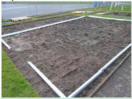
On the left you can see the steel base has all been set out before it is all fixed together.. From this base the rest of the framework is then assembled...........
