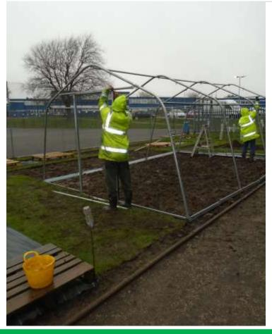
Once the steel framework has all been fitted together, the whole structure is fixed into the ground with steel posts to give it excellent ground anchorage... A vital component of the poly tunnel set up especially bearing in mind some of the extremely high winds we have been experiencing in recent times.......
